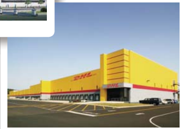
DHL Central Data Center
