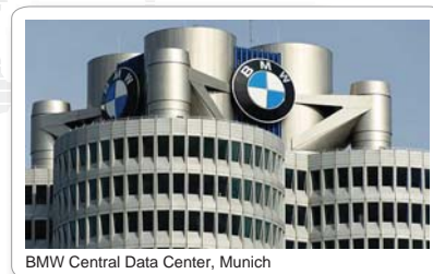
BMW Central Data Center, Munich
