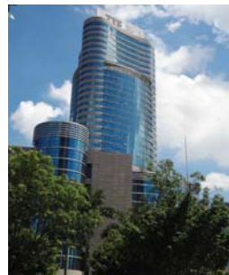
ZTE Central Office, Shenzhen
